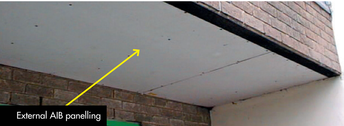
AIB soffit board
